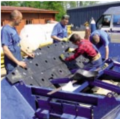
Low weight makes installation of WT7000 liner parts easy.
